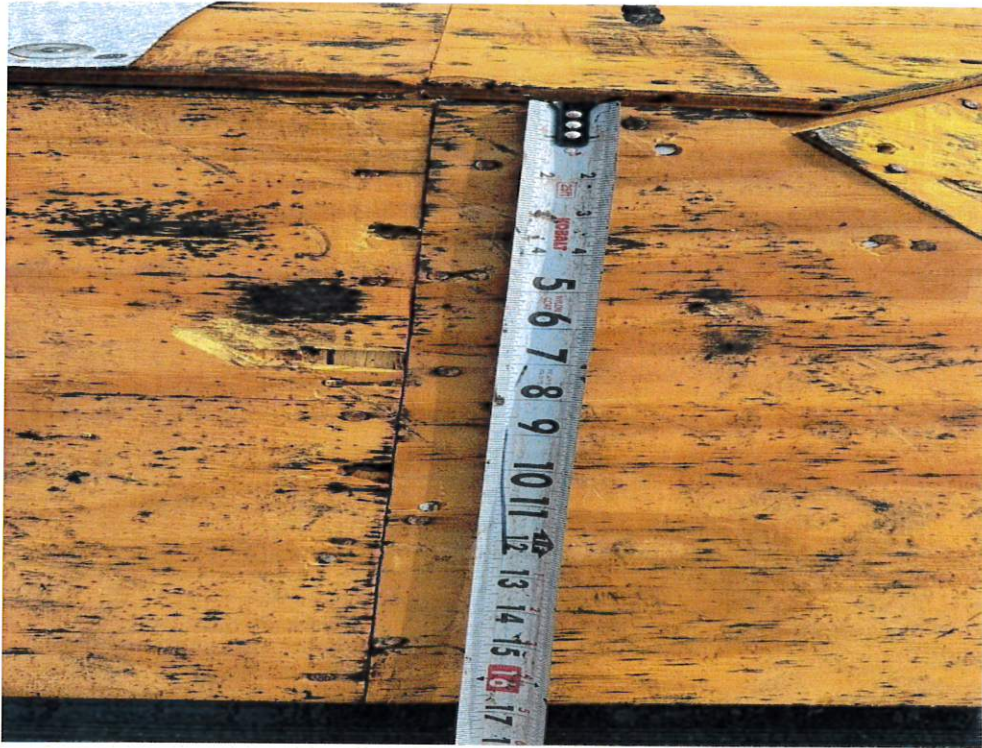
Figure 3 – Sheathing Fastener Spacing
