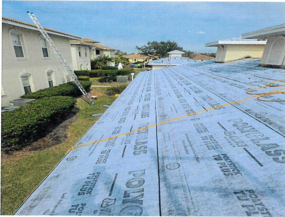
Figure 7 – Secondary Water Resistance
