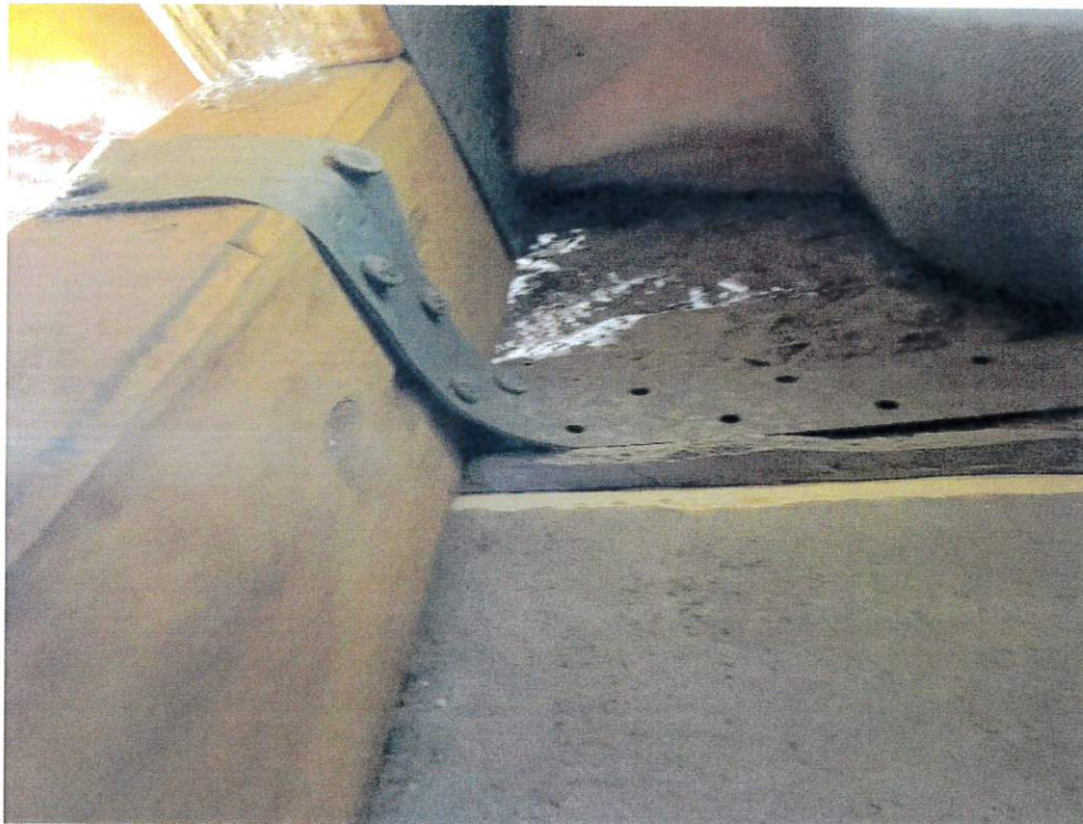
Figure 6 - Roof to Wall Attachment
