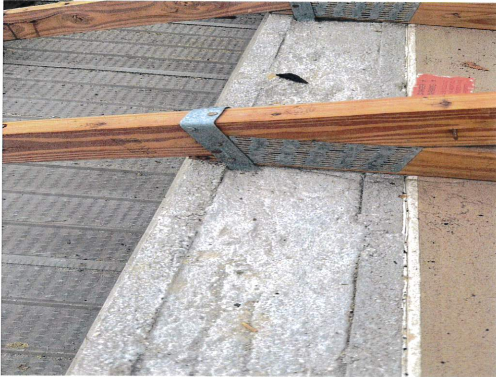
Figure 5 – Roof to Wall Attachment
