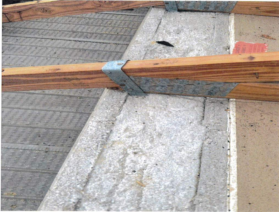
Figure 5 – Roof to Wall Attachment
