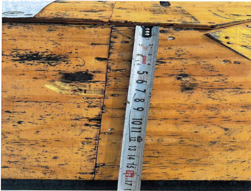
Figure 3 – Sheathing Fastener Spacing
