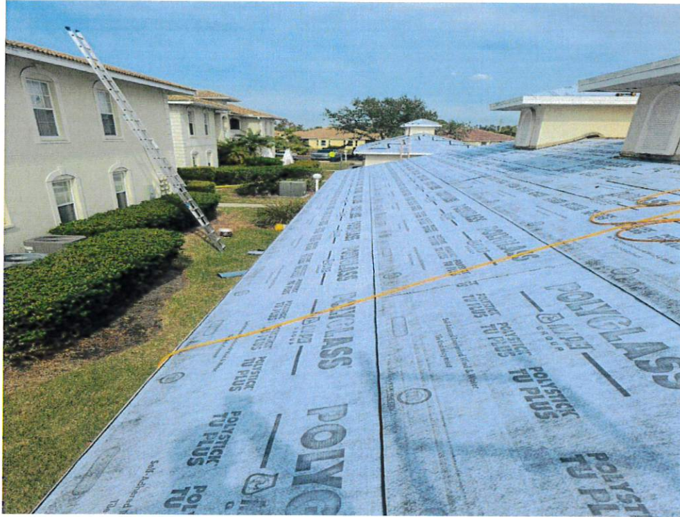
Figure 7 – Secondary Water Resistance
