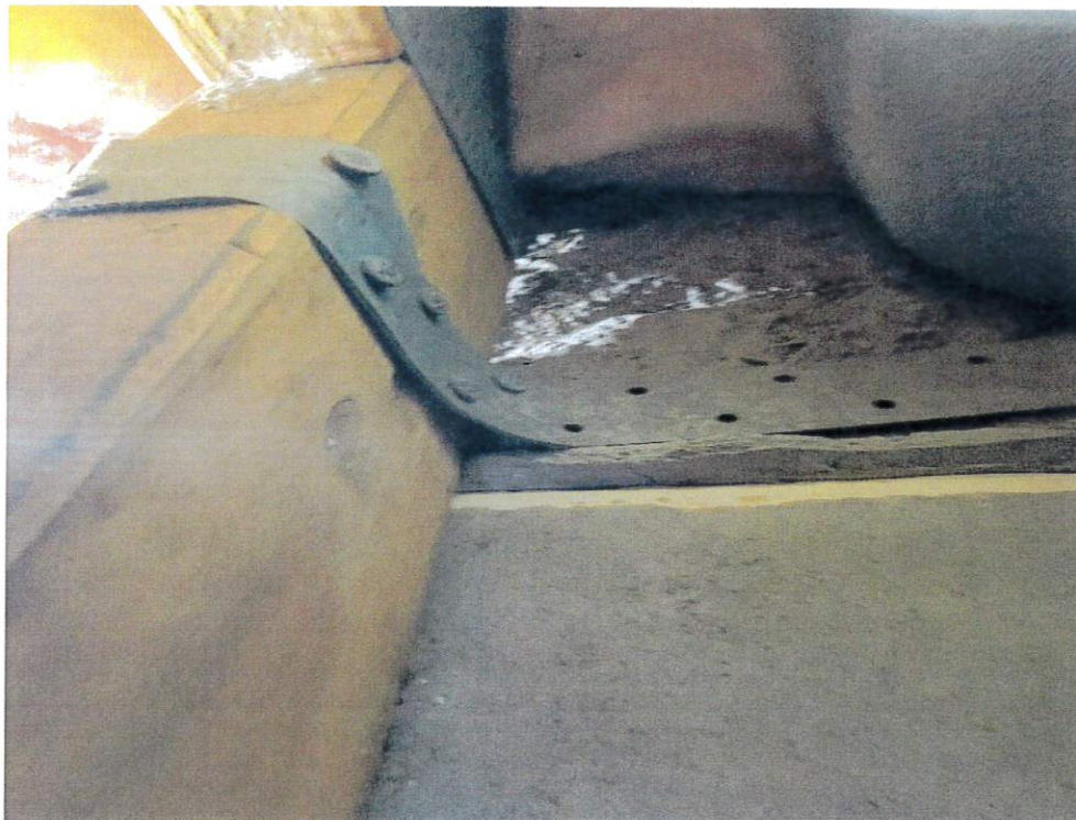
Figure 6 - Roof to Wall Attachment
