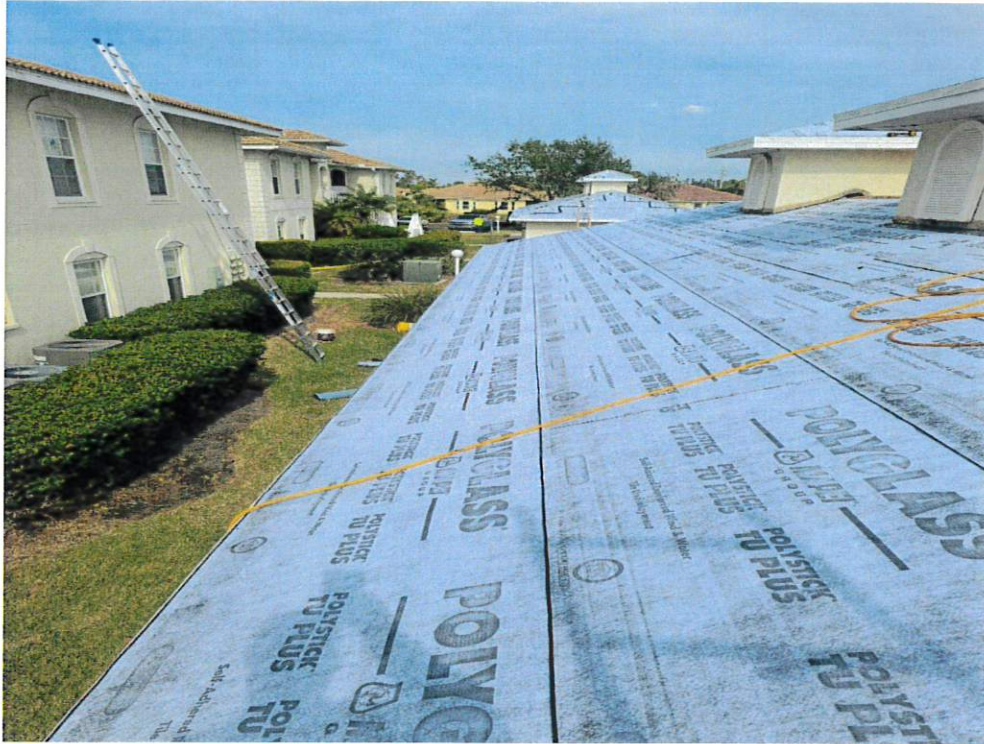
Figure 7 – Secondary Water Resistance
