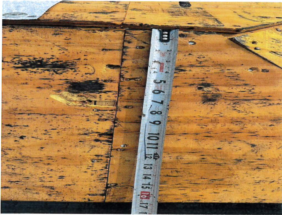
Figure 3 – Sheathing Fastener Spacing
