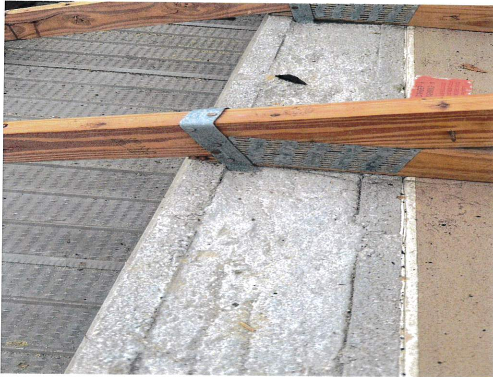
Figure 5 – Roof to Wall Attachment
