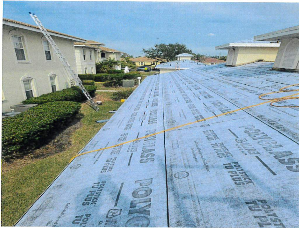
Figure 7 – Secondary Water Resistance
