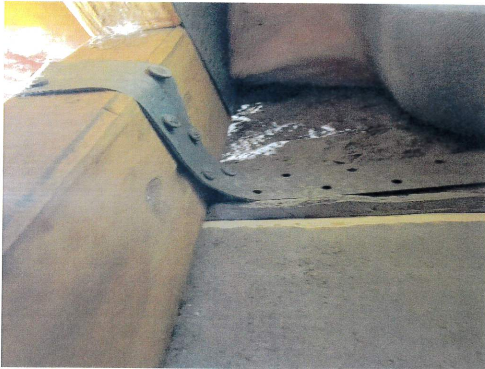
Figure 6 - Roof to Wall Attachment
