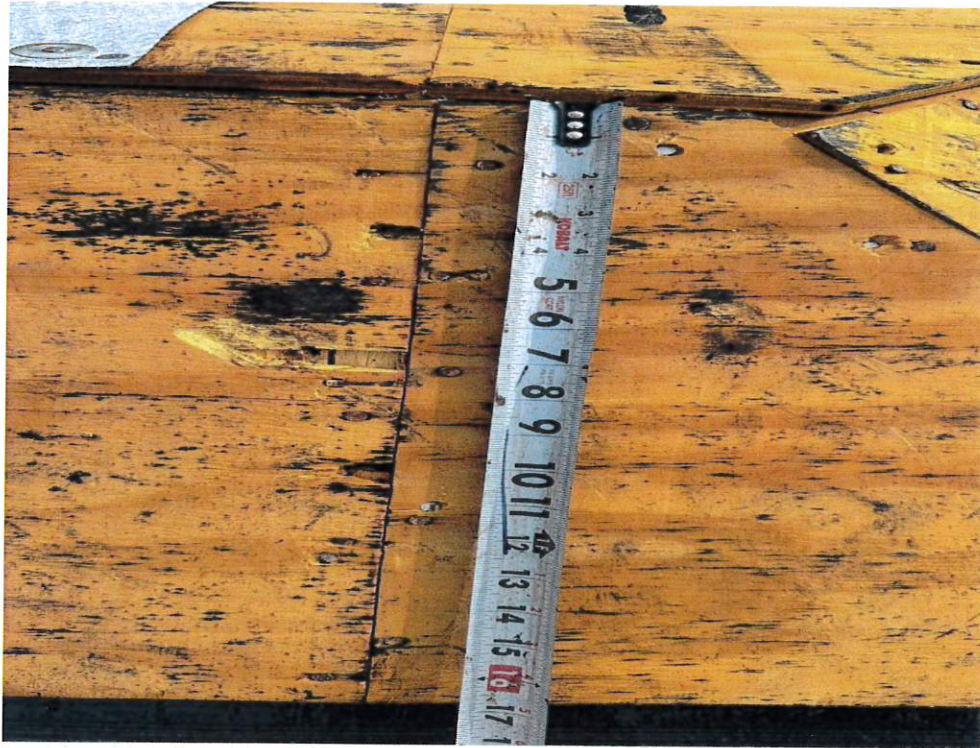
Figure 3 – Sheathing Fastener Spacing
