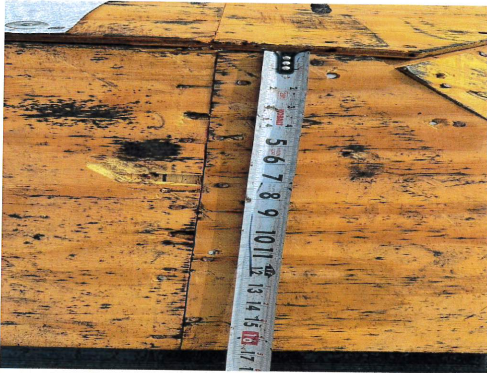
Figure 3 – Sheathing Fastener Spacing
