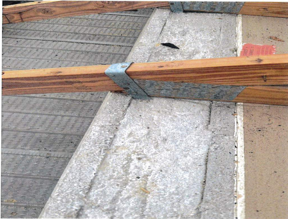
Figure 5 – Roof to Wall Attachment
