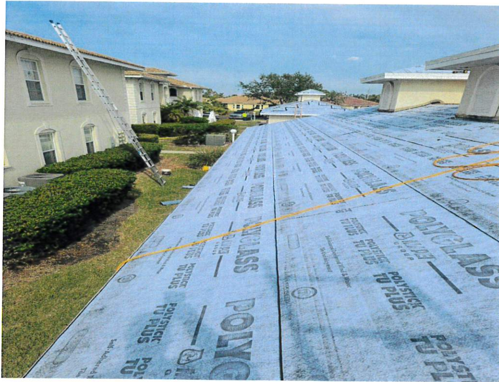
Figure 7 – Secondary Water Resistance
