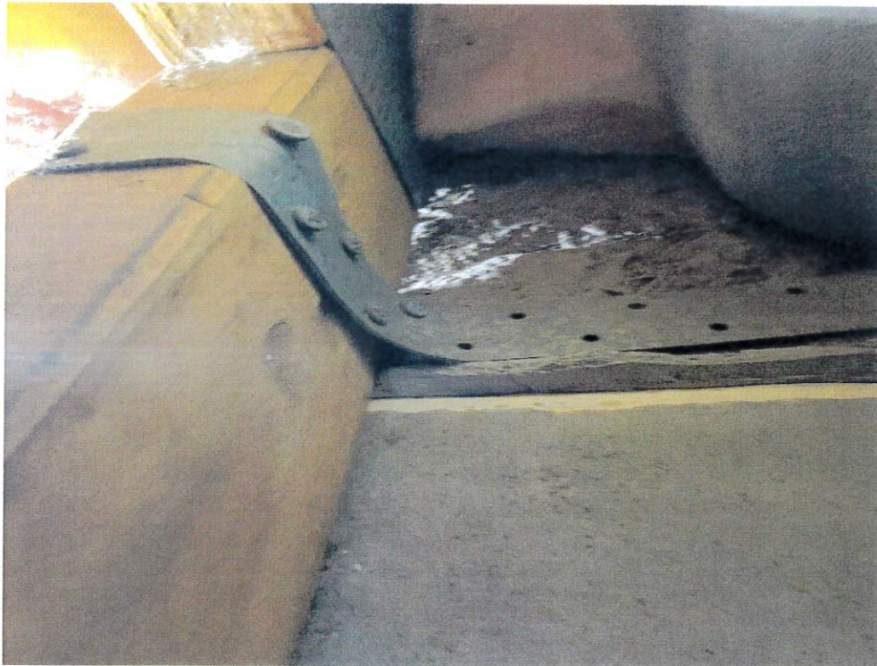
Figure 6 - Roof to Wall Attachment
