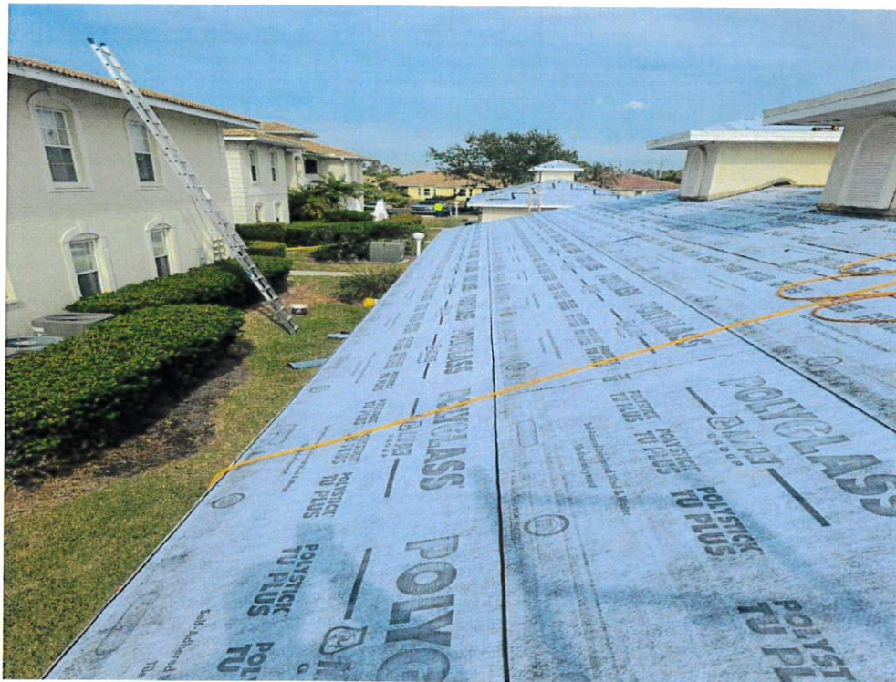
Figure 7 – Secondary Water Resistance
