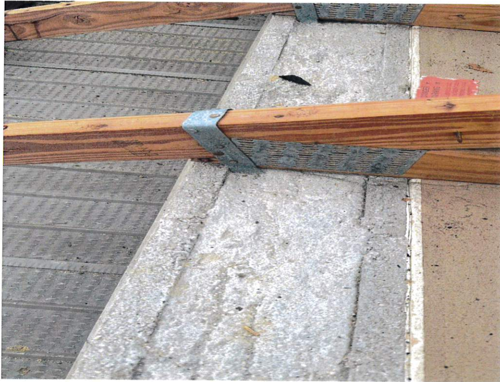
Figure 5 – Roof to Wall Attachment
