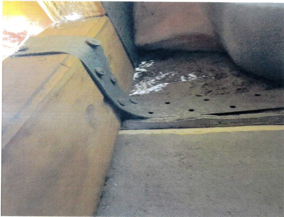
Figure 6 - Roof to Wall Attachment
