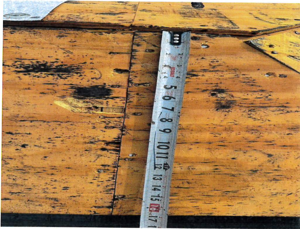
Figure 3 – Sheathing Fastener Spacing
