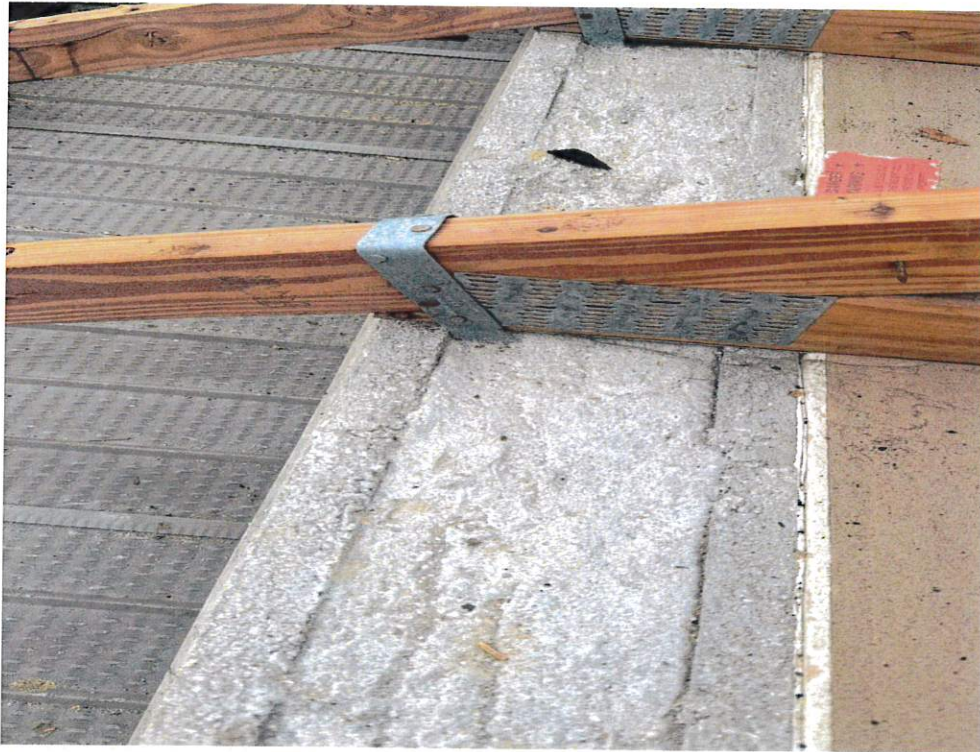
Figure 5 – Roof to Wall Attachment
