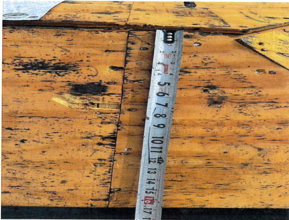
Figure 3 – Sheathing Fastener Spacing
