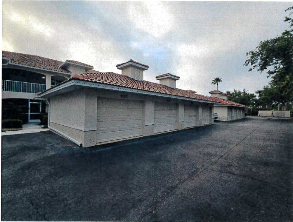
Figure 1: Roof Type (Concrete Barrel Tile) and Geometry (Hip)
