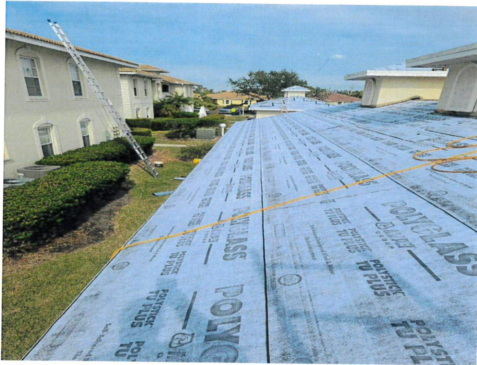
Figure 7 – Secondary Water Resistance
