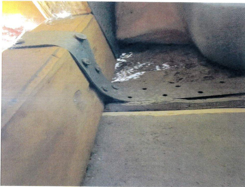
Figure 6 - Roof to Wall Attachment
