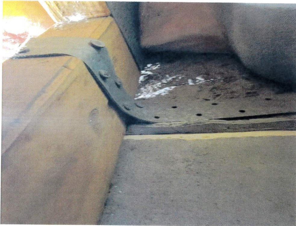
Figure 6 - Roof to Wall Attachment
