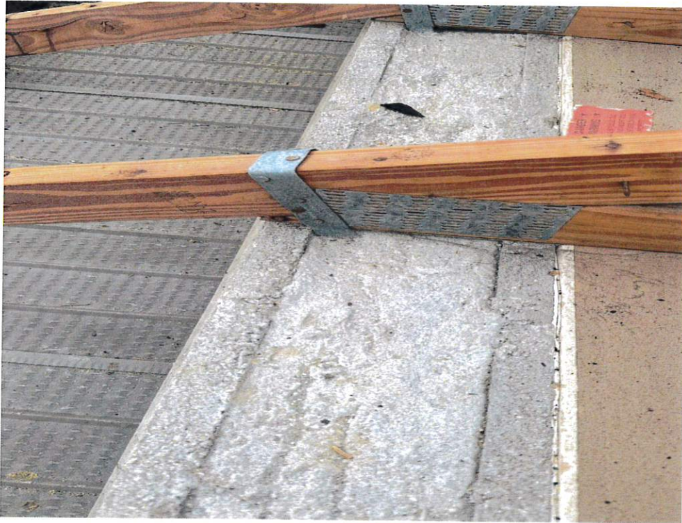
Figure 5 – Roof to Wall Attachment
