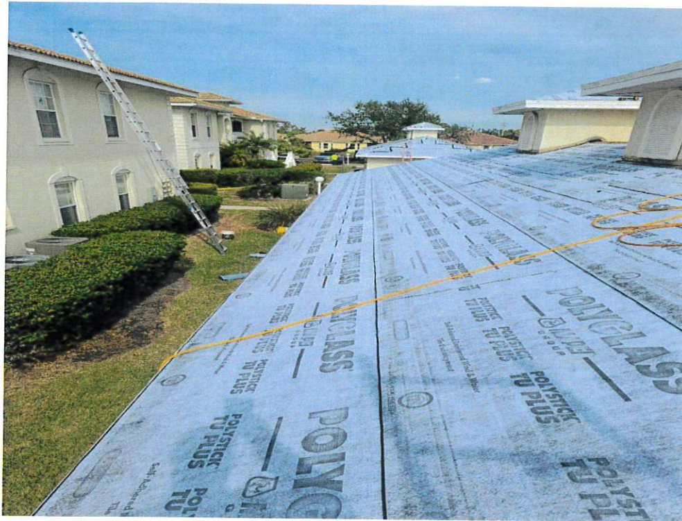
Figure 7 – Secondary Water Resistance
