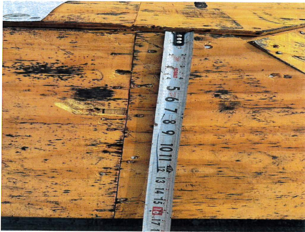
Figure 3 – Sheathing Fastener Spacing
