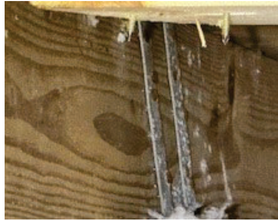
Roof to Wall: Wrap with 3+ Nails
