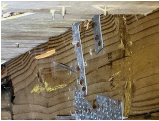
Roof to Wall: Wrap with 3+ Nails
